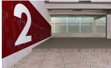
Parking garage reinforcement
